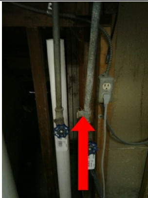
Galvanized water piping present. No visible corrosion observed.
