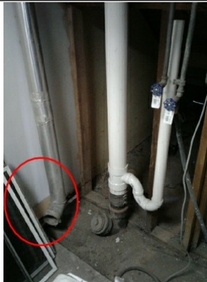
Exhaust for a future dryer, recommend cleaning dryer vent.
