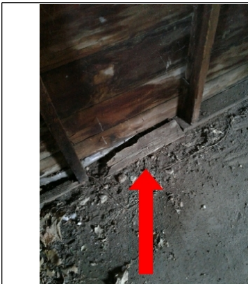
Sill plates were deteriorated in multiple areas.
