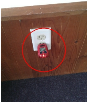
Electrical receptacles in the porch area had reverse polarity. Recommend repair.
