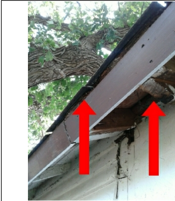
More deterioration observed on soffit and roof.
